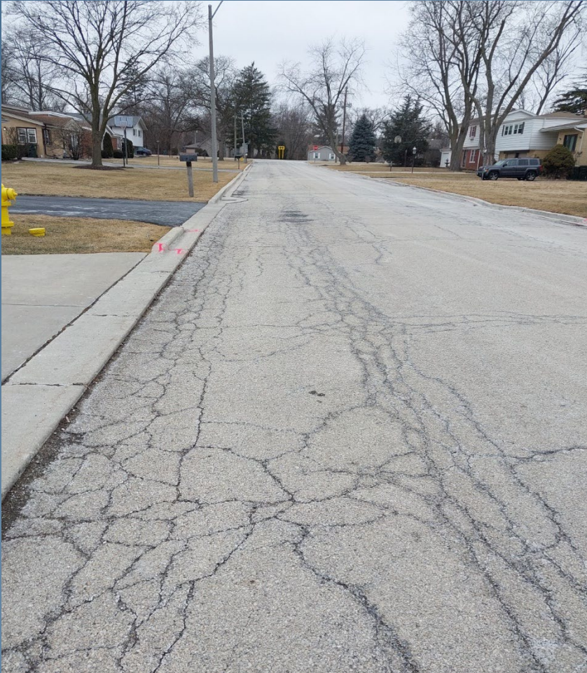
TERRY LANE FACING WEST
